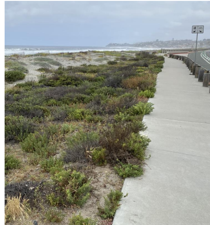
Vegetated dunes with buried cobble berm adjacent to Coast Highway along Cardiff State Beach
