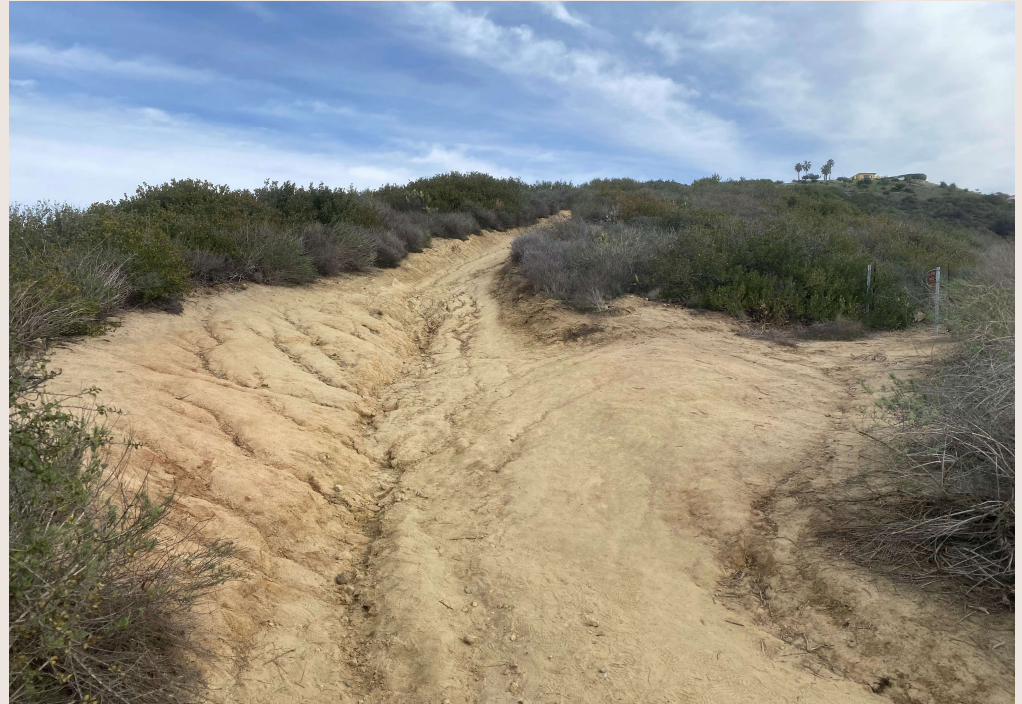
Poorly designed trails concentrate runoff, resulting in channelization and widening
