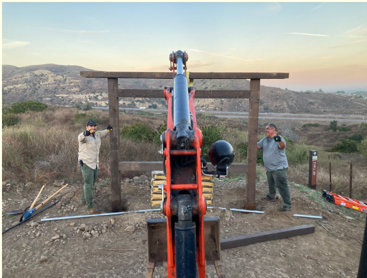
Kiosk Installation by OC Parks Maintenance Team
