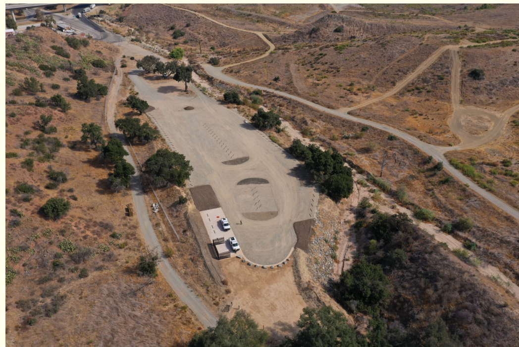
Parking and Staging Area for Gypsum Canyon Wilderness in 2021
