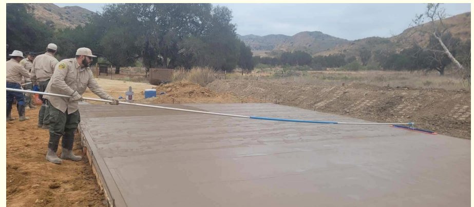
Parking and Staging Area installation of new concrete ADA parking pads
