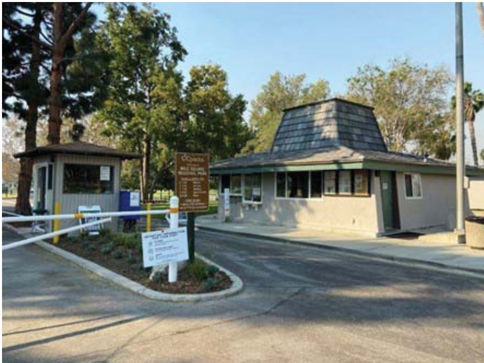
Photo 2: View of the Existing Ranger Station Built Structure located in the north east end of MISQ
