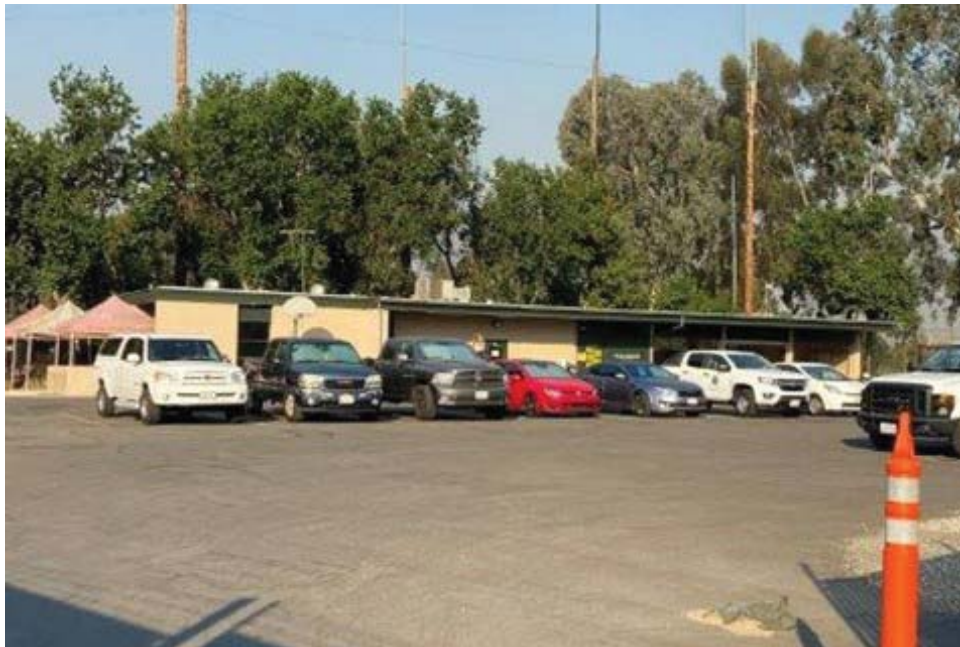
Photo 4: View of the western garage in maintenance yard, primary elevation, west
