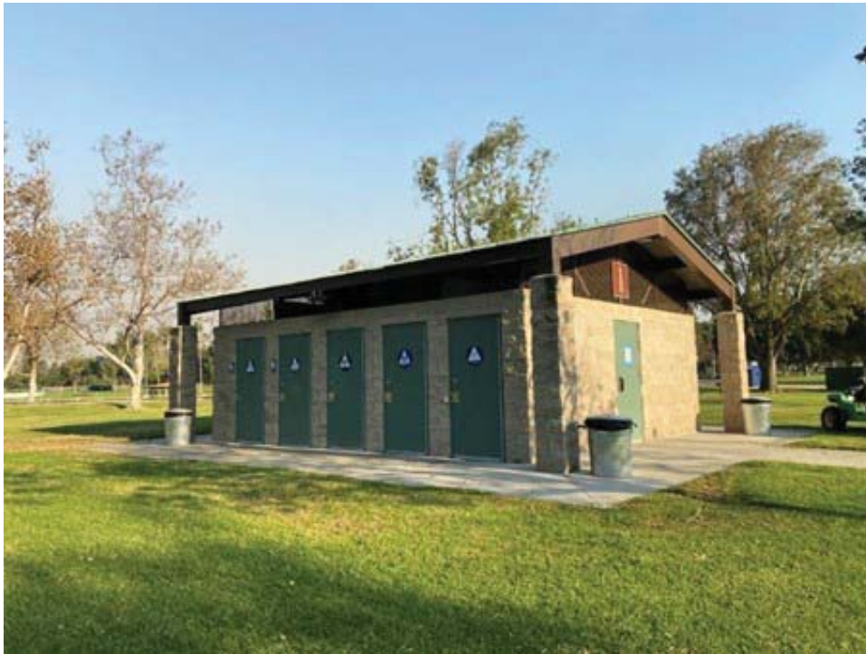
Photo 1: View of the restroom building, facing northwest
