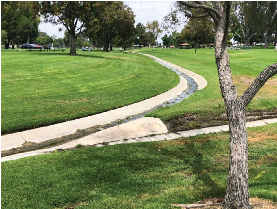
Photo 3: View of stormwater drainage channel located in the south end of MISQ.
