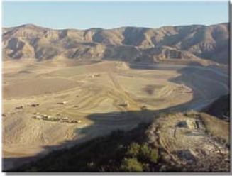
Aerial Photo Olinda Alpha Landfill
