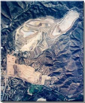
Aerial Photo Olinda Alpha Landfill
