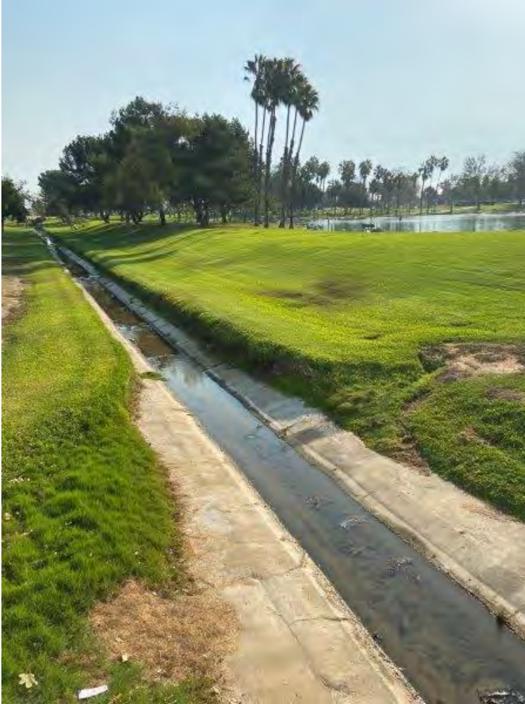
Exhibit 11. Concrete flood control channel, camera facing north.
