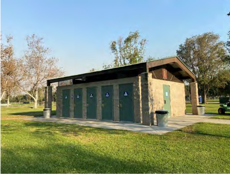
Exhibit 4. Restroom building, design one, camera facing west northwest.
