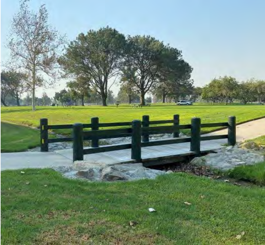
Exhibit 12. Pedestrian bridge over channel, camera facing south.
