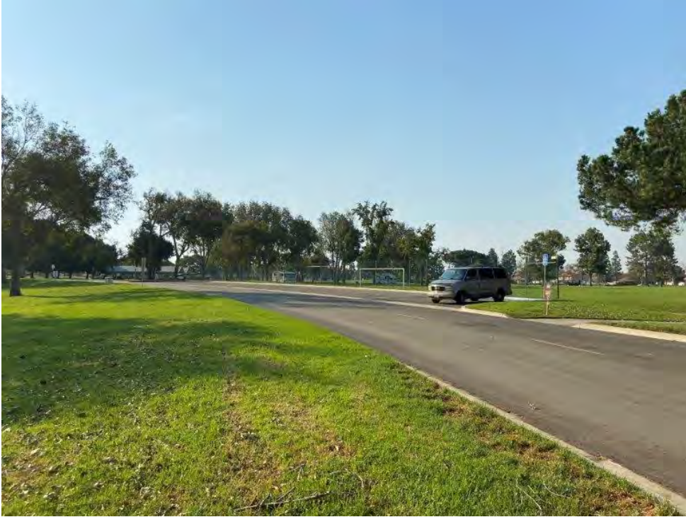
Exhibit 20. Non-original roadway expansion for parking in center of park, camera facing southeast.
