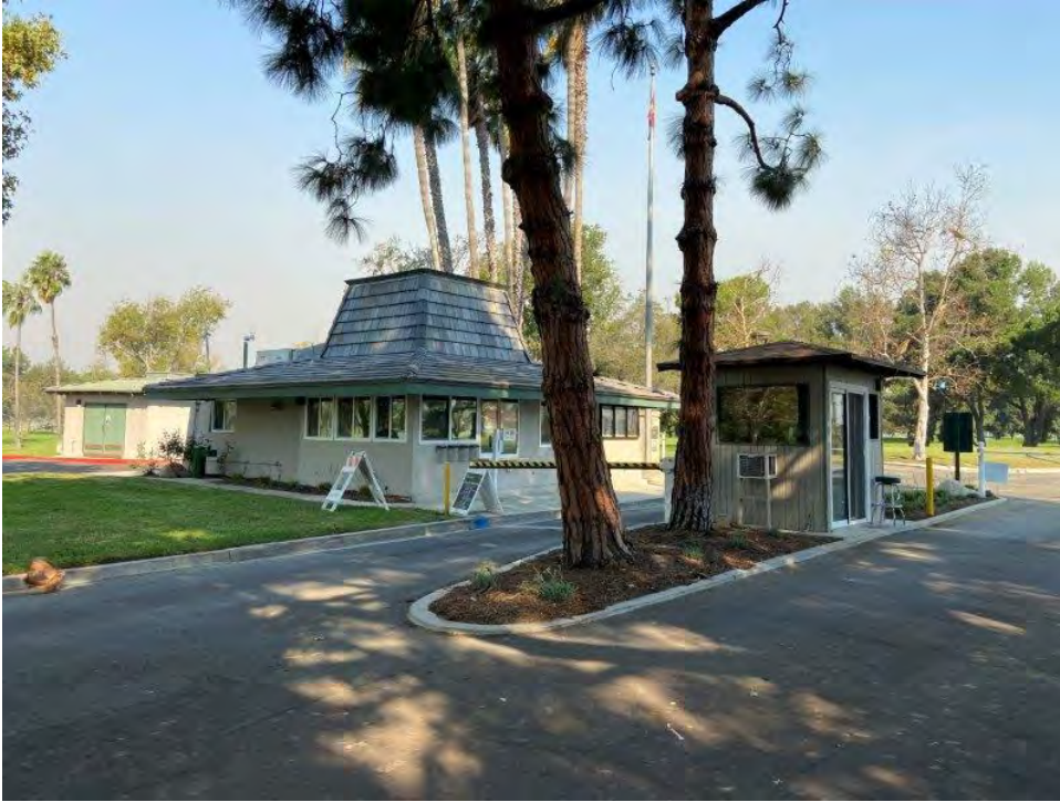
Exhibit 8. Administrative ranger building and fee booth, camera facing northwest.
