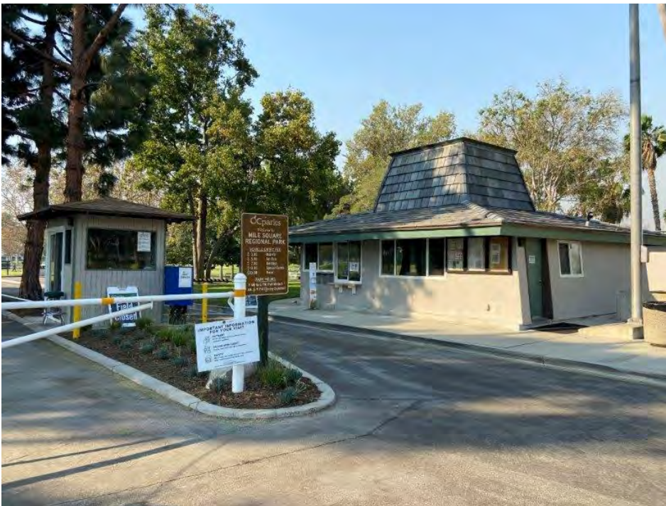
Exhibit 7. Administrative ranger building and fee booth, primary elevation camera facing southwest.
