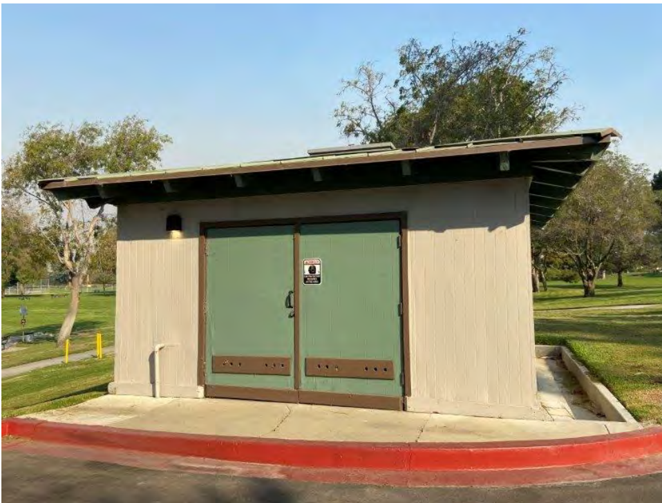
Exhibit 9. Utility shed at ranger station complex, south elevation, camera facing north.
