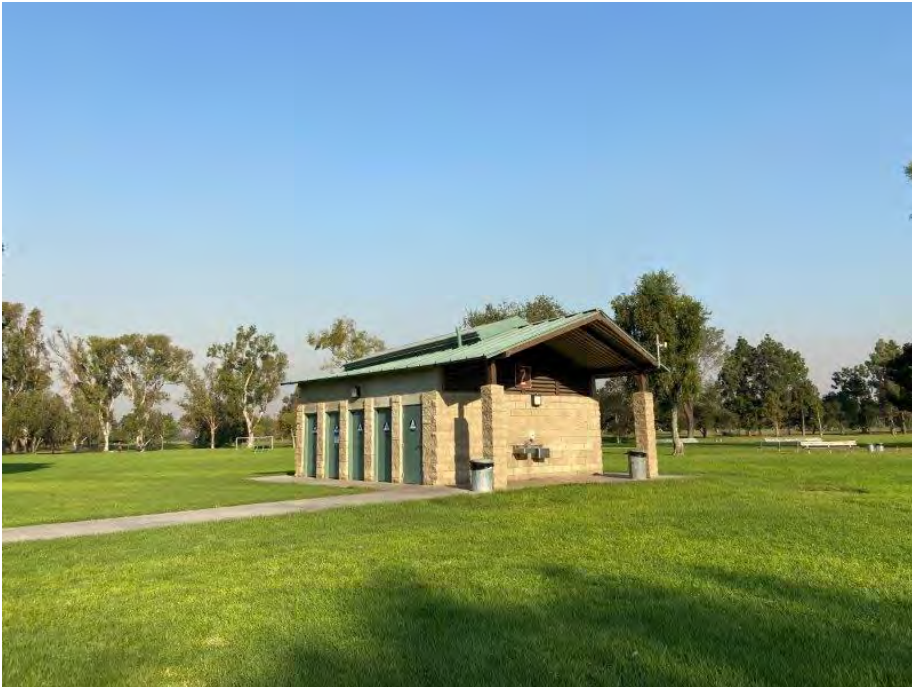
Exhibit 5. Restroom building, design two, camera facing northwest.
