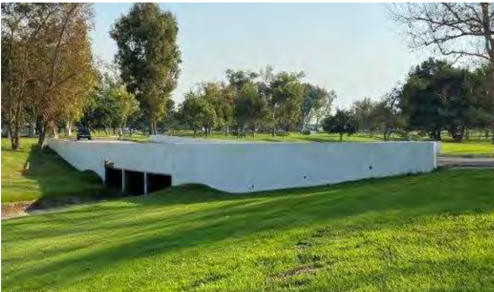
Exhibit 13. Automobile bridge over flood control channel, southwest elevation, camera facing northeast.
