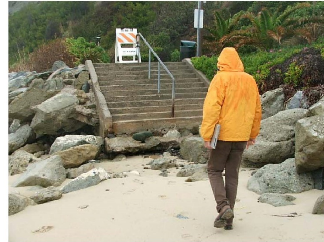
PHOTO 1-EXISTING NORTHERLY ACCESS STAIR
