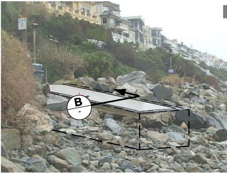
EXISTING SOUTH ACCESS RAMP- NORTH RAMP AND NORTH STAIRS SIMILAR
