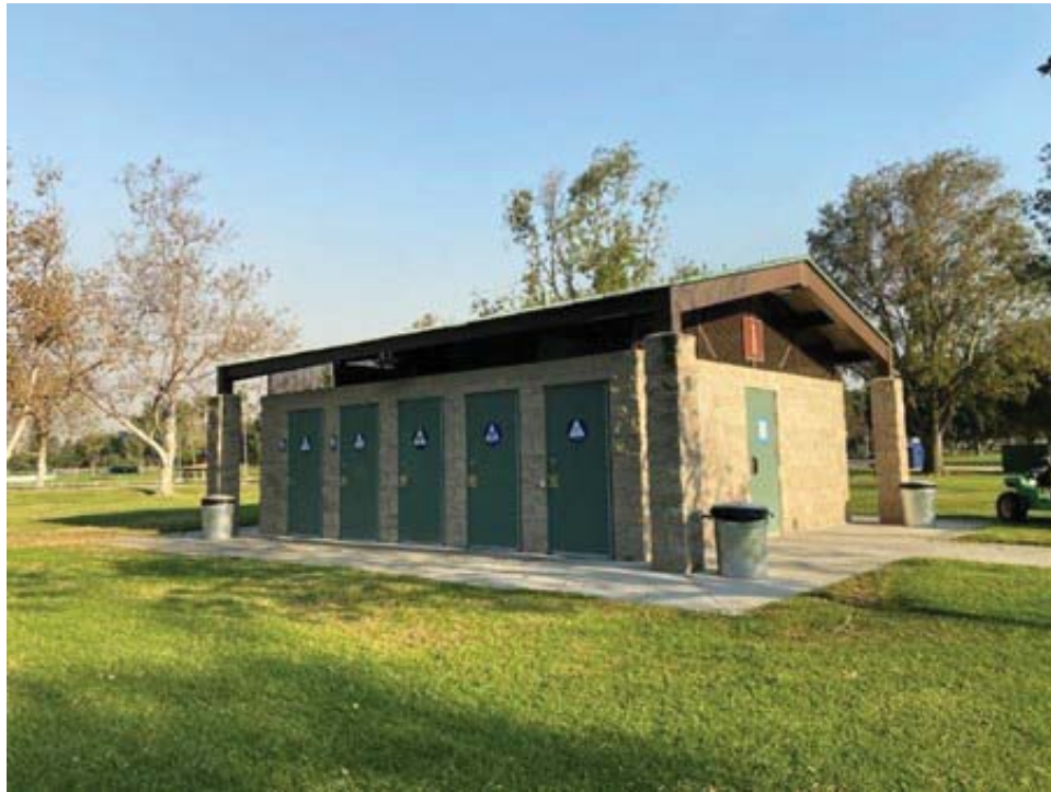
Photo 1: View of the restroom building, facing northwest
